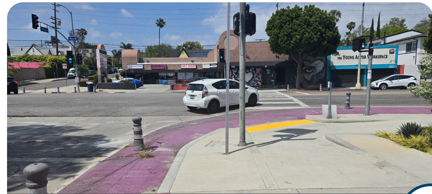
Pico Boulevard Great Streets Pedestrian Bulb-outs (Image Courtesy of LADOT)
